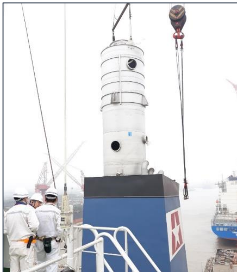
The new scrubber tower during descent in the existing funnel at the yard
