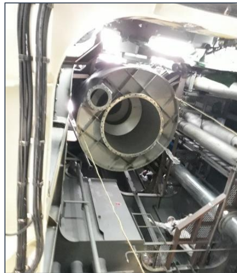
The new scrubber tower during descent - view from inside the funnel
